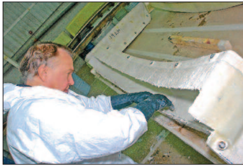
Michael Haley working on a ventilation duct for one of the capsules on the London Eye
