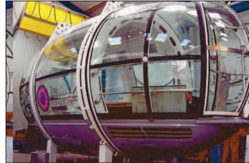
Quantum is making replacement panels as part of the refurbishment of the London Eye's capsules
